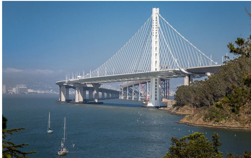
The New East Span of the San Francisco Oakland Bay Bridge
