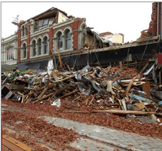
Damage to masonry building, 2011
